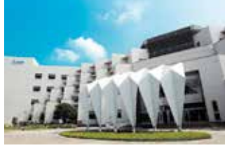
Tainan Plant (Diamond-rated Green Building)
